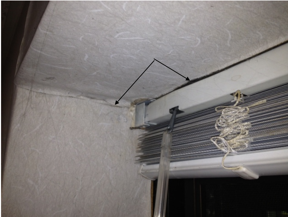
Wallpaper barely hanging on. Mold growth observed right under creases.
