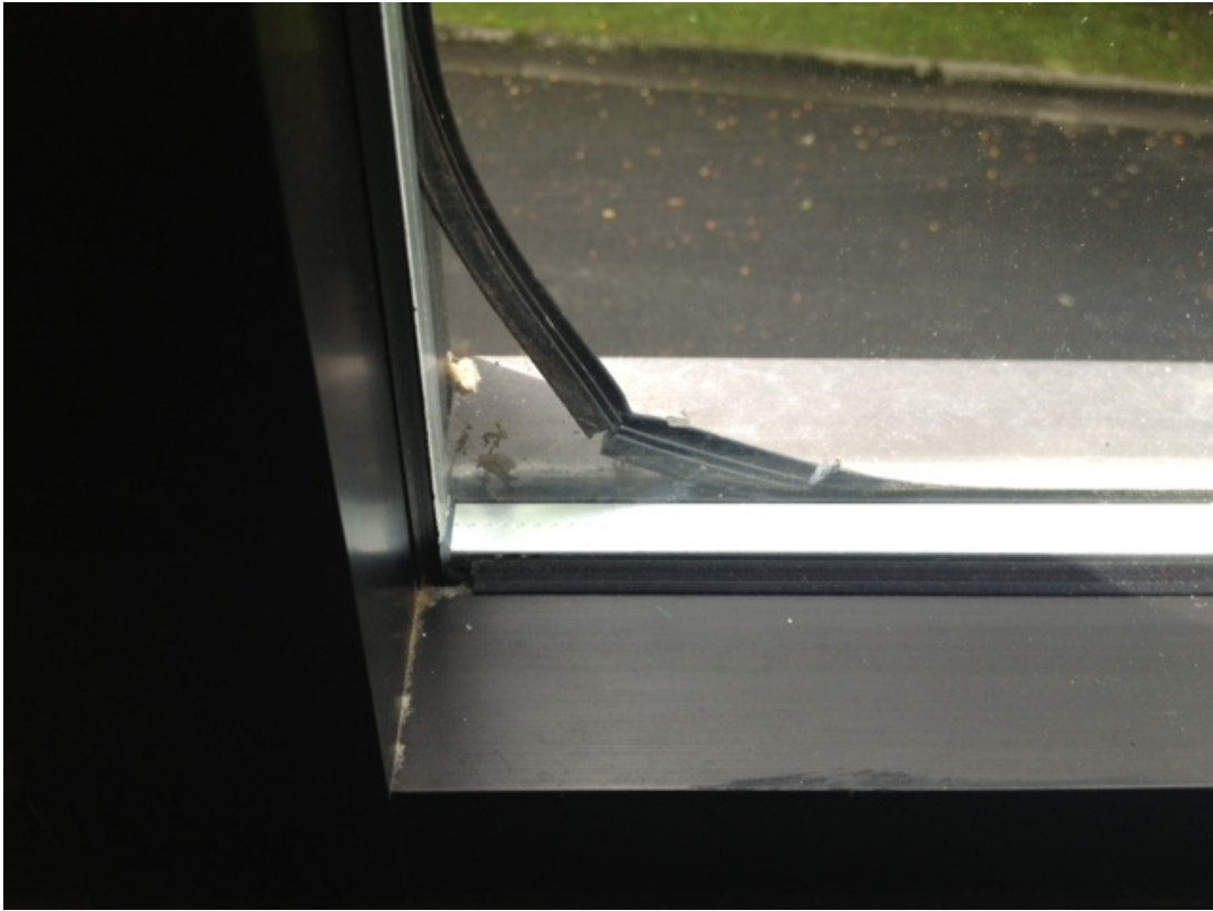
Exterior seals coming apart around the window.
