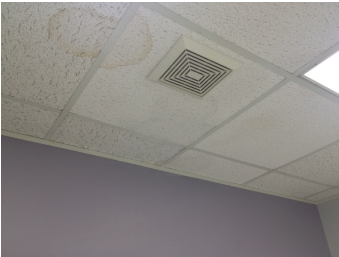
Exam Room 4: Separate issue of leaky ductwork and/or drain pan above ceiling.
