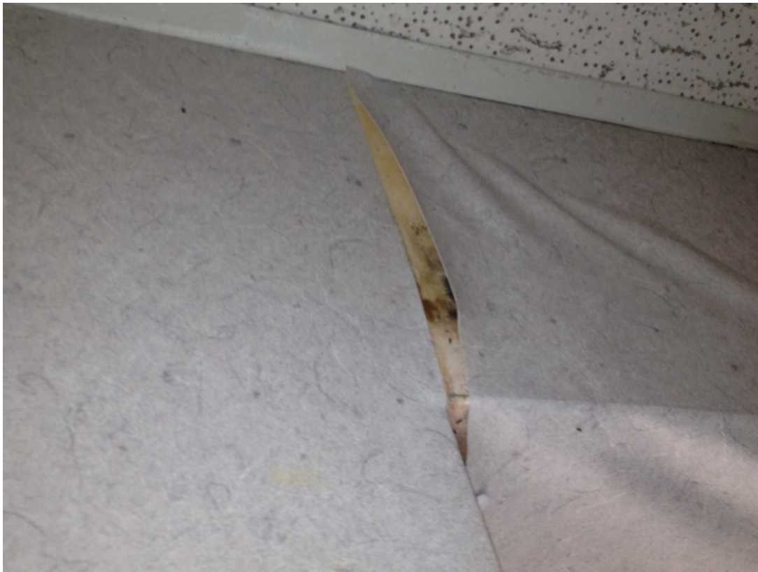
Above the upper left corner of lobby windows; visible mold growth seen forming under the wallpaper.
