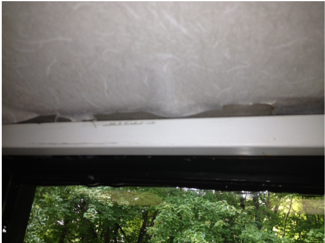
Close up view of vacant back office, top of windows. Wallpaper coming unglued from moisture and mold growth behind.
