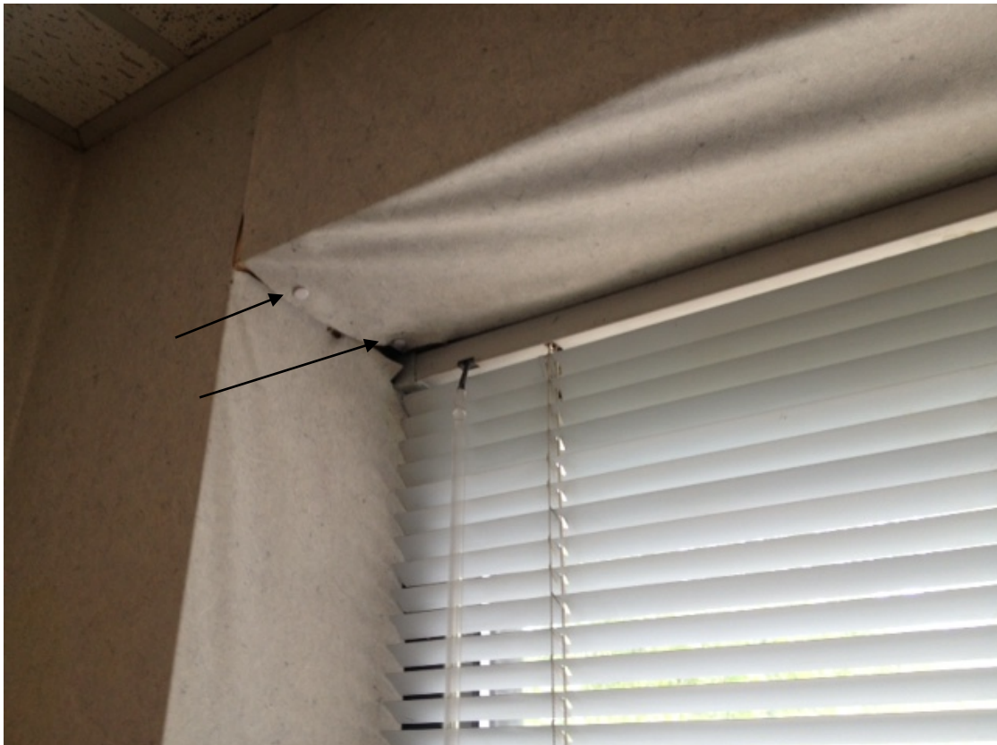
Wallpaper around windows affected from moisture intrusion, being held in place by thumbtacks.
