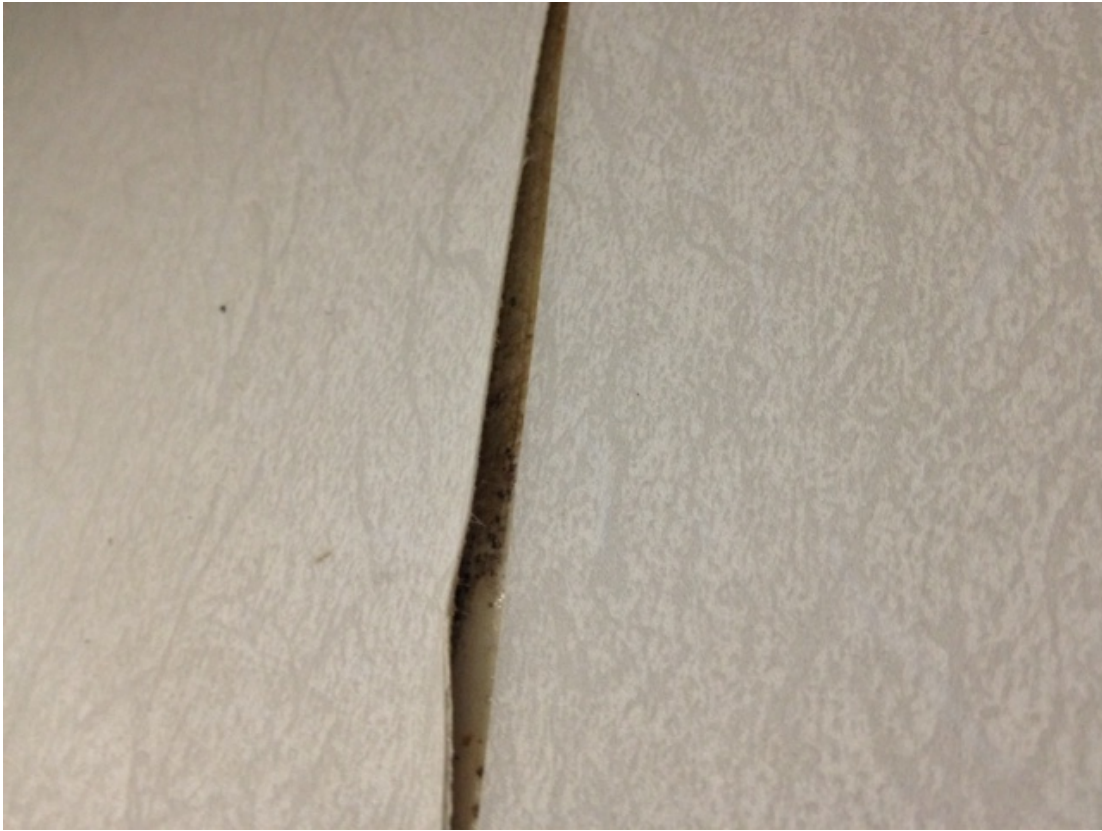
Seam in wallpaper coming apart in back office area exterior wall; visible mold growth evident behind it.
