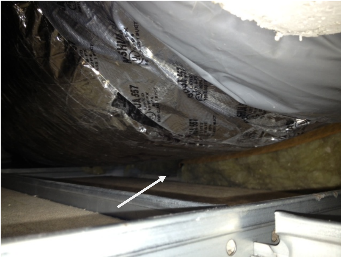
Dirty insulation, or mold growth from wicking up moisture? Unsure; could not reach.
