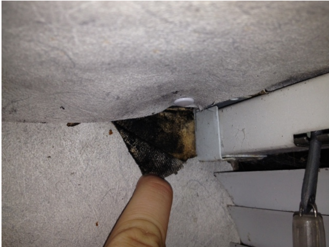
Inside window casing, upper left corner of lobby windows. Visible mold growth heavy behind the wallpaper.
