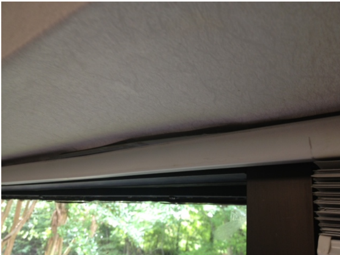
Vacant back office area, same issue with wallpaper coming unglued because of moisture and subsequent mold growth behind it.
