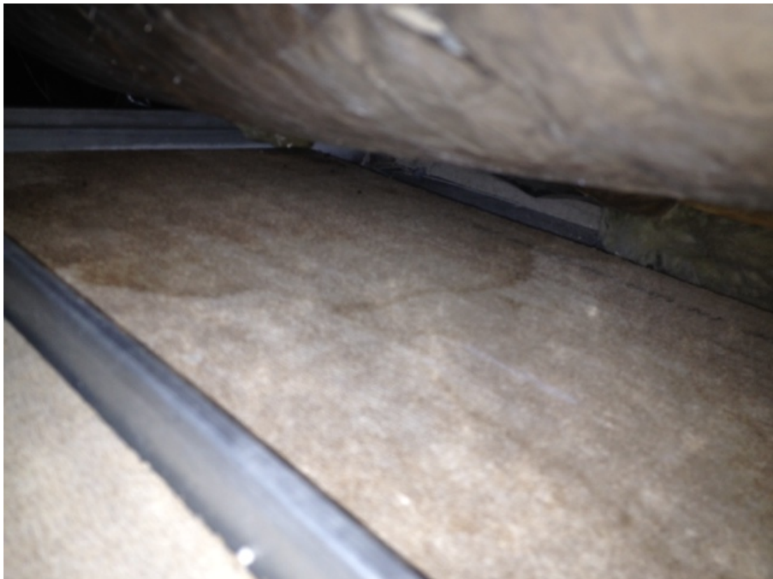
Good view of where moisture leaks above ceiling tiles in Exam Room 4 has taken place.
